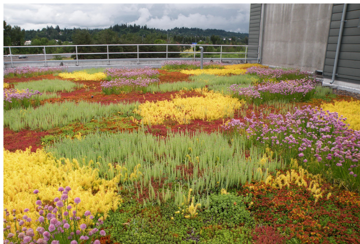
Installed vegetated roof assembly
